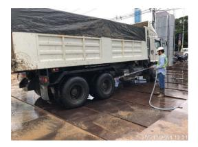
1.2 Spray water on the construction area or the activity area affected by construction dust dispersal at least twice a day (morning and afternoon) and during dry weather, or as appropriate to the climate. Ensure that the soil surface is kept wet to prevent dust dispersal and minimize the impact on neighboring communities.
