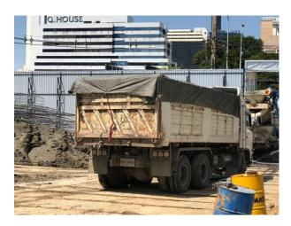
5.4 Tires of transport vehicles leaving the construction area must be washed each time to prevent debris, sand, and dirt from being deposited on public roads.
