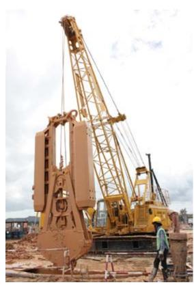
polymer) is filled to protect the excavated trench against soil collapse. After that, a steel cage is installed and a concrete is poured into the trench. After the concrete has set and reached the required strength, the underground excavation will be performed as well as the construction of underground structures.
