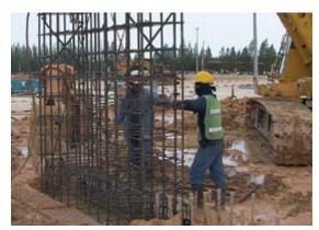
A barrette pile is constructed by excavating the soil in accordance with the required cross section size and depth. A stabilizing slurry (bentonite and polymer) is added to protect the borehole against soil collapse. After excavation, a steel cage is installed and a concrete is poured.
