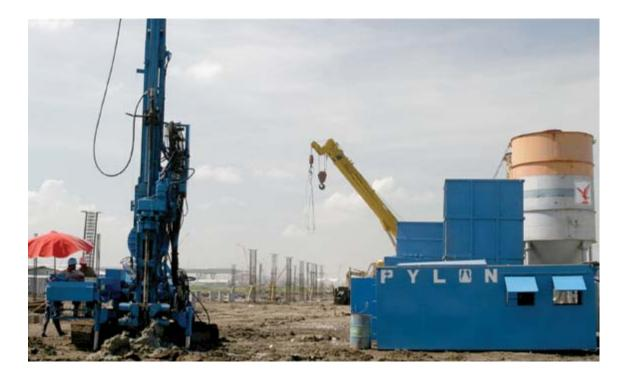
The objective of ground improvement is to strengthen the existing soil structure which can lead to the increase of soil bearing capacity and prevention of lateral soil movement. The Company provides this type of service by injecting cement grout at a high pressure between 200 to 400 bars. Type of work can be categorized as follows:
