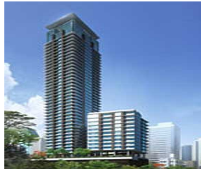
Amanta Condo Rama4 Bored Piles
