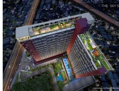
Privacy Rama9 Bored Piles
