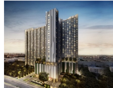
Buddha Port Bored Piles
