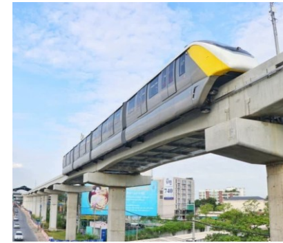
MRT Yellow & Pink Line Bored Piles / Barrette Pile
