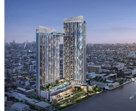
Wan Vela Bored Piles
