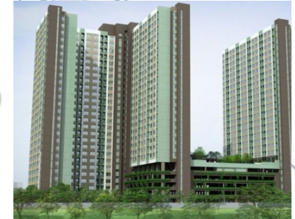
L.P.N. Ville Nakorn In Bored Piles
