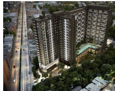
Parkland Phetkasem-Taphra Bored Piles
