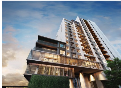
Parkland Charan Bored Piles
