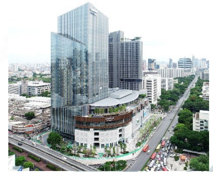
Samyarn Mitrtown Bored Piles / D-Wall
