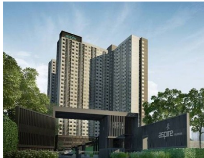
Aspire Erawan Bored Piles
