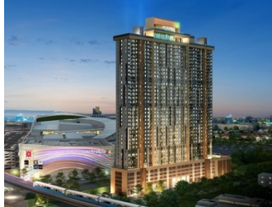
Plum Condo Ph.1-2 Bored Piles
