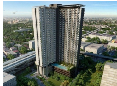
Parkland Ratchada- Wongsawang Bored Piles
