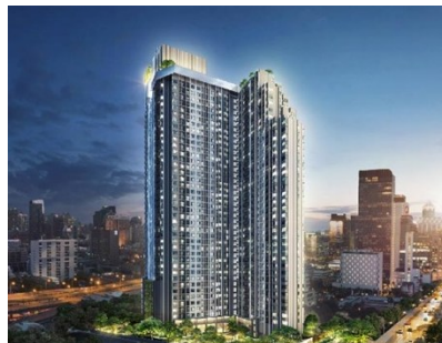
Life on wireless Bored Piles
