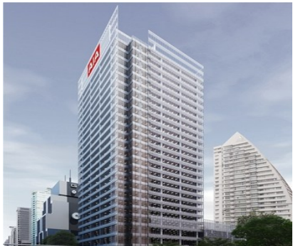
AIA - Sathorn Bored Piles
