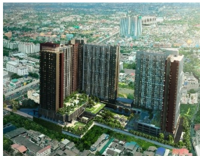
Parkland Phetkasem56 Bored Piles
