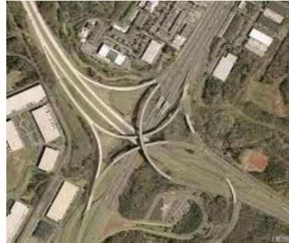
South Interchange Bored Piles
