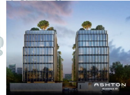
Ashton Residence 41 Bored Piles
