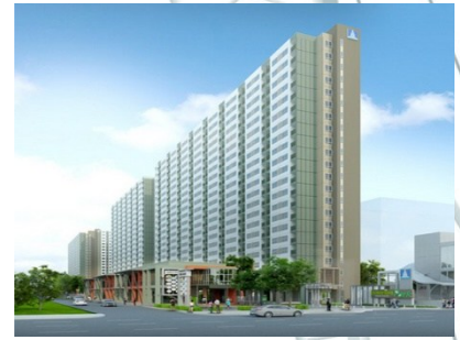
L.P.N. Phetkasem 98 Bored Piles
