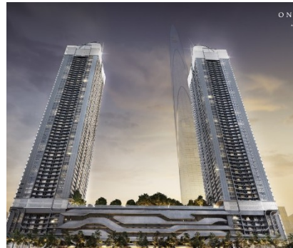
One9Five Rama9 Bored Piles
