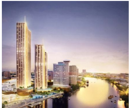
The ICONSIAM Bored Piles / Jet Grouting
