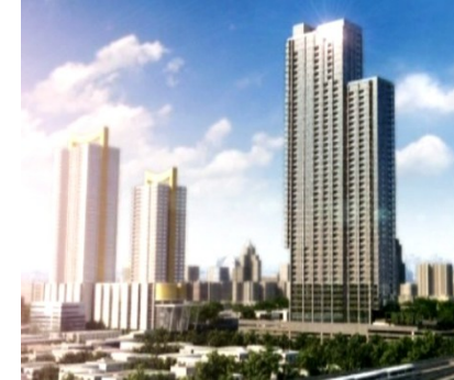
Circle Living Prototype Bored Piles
