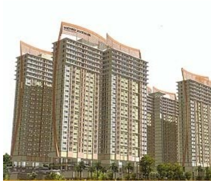
Metro Avenue Bored Piles
