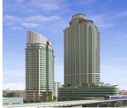
Le Luk Condo (A+B) Bored Piles
