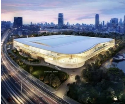
Queen Sirikit National Convention Center Bored Piles / Pile walls / D-Wall
