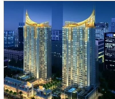
TC Green I/II Bored Piles
