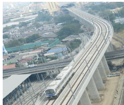
Airport Rail Link Bored Piles
