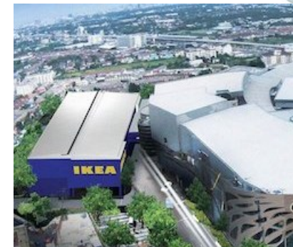
IKEA Westgate Bored Piles
