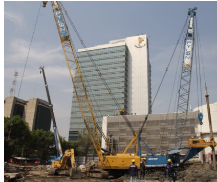
EGAT Car park & HQ Bored Piles / Constructions
