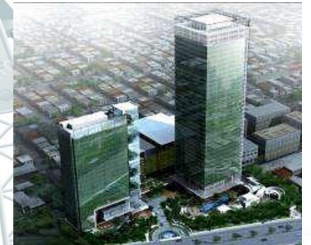
AIA - CMC Bored Piles
