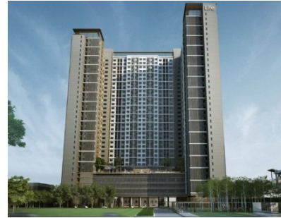
Life Asoke Bored Piles
