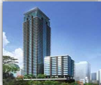
Amanta Condo Rama4 Bored Piles
