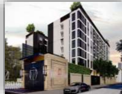
Maestro07 Bored Piles
