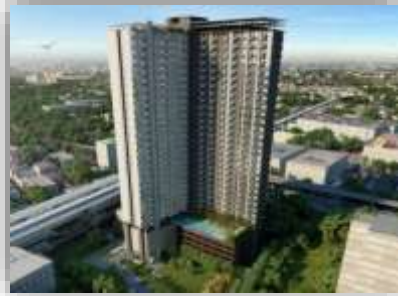
Parkland Ratchada- Wongsawang Bored Piles
