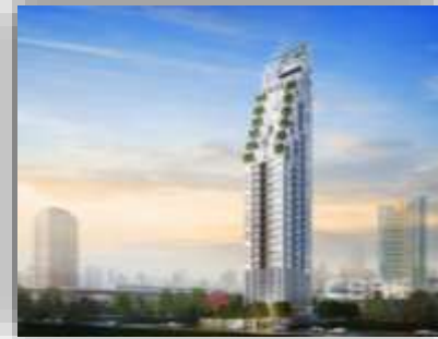
Muniq SK23 Bored Piles
