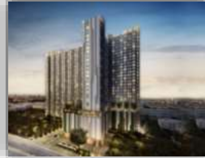
Buddha Port Bored Piles
