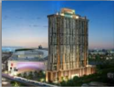
Plum Condo Ph.1-2 Bored Piles
