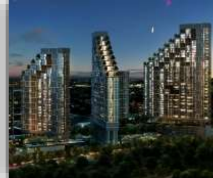
The One Residence Bored Piles
