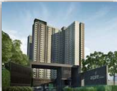
Aspire Erawan Bored Piles
