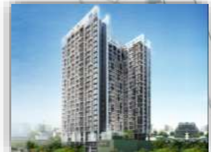
IDEO Mobi Rama 9 Bored Piles
