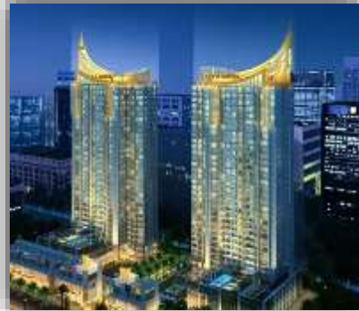
TC Green I/II Bored Piles
