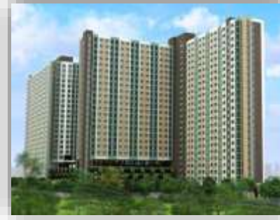
Lumpini Park Rama9 Bored Piles
