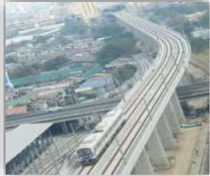
Airport Rail Link Bored Piles
