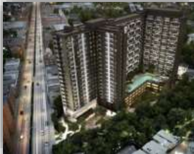
Parkland Phetkasem-Taphra Bored Piles
