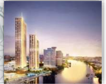
The ICONSIAM Bored Piles / Jet Grouting
