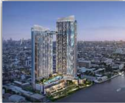
Wan Vela Bored Piles
