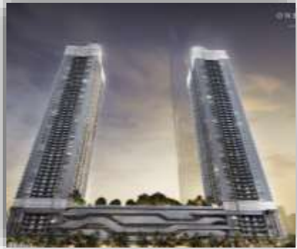
One9Five Rama9 Bored Piles
