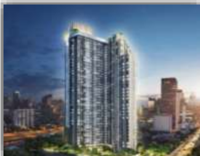
Life on wireless Bored Piles
