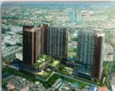
Parkland Phetkasem56 Bored Piles
