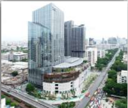
Samyarn Mitrtown Bored Piles / D-Wall
