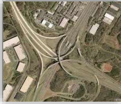
South Interchange Bored Piles
