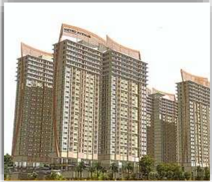
Metro Avenue Bored Piles
