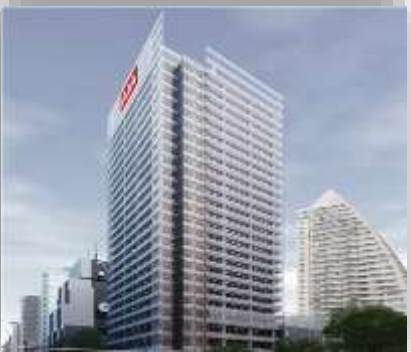
AIA - Sathorn Bored Piles
