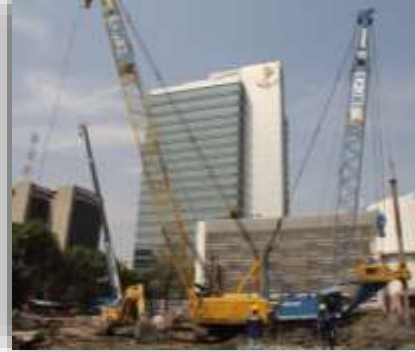
EGAT Car park & HQ Bored Piles / Constructions
