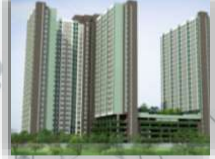
L.P.N. Ville Nakorn In Bored Piles
