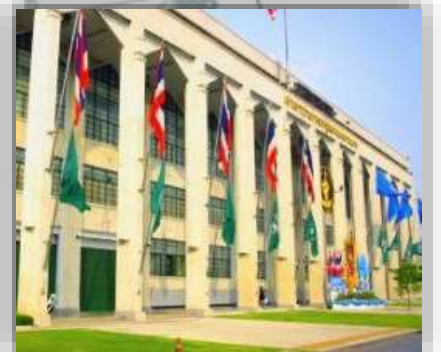
BMA Building Bored Piles
