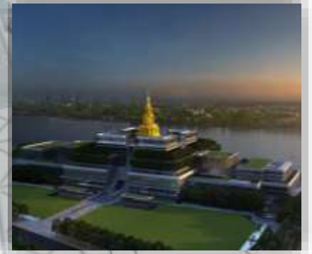
Thai National Assembly Bored Piles
