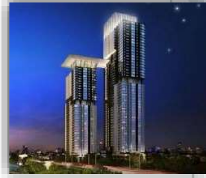
Starview Bored Piles
