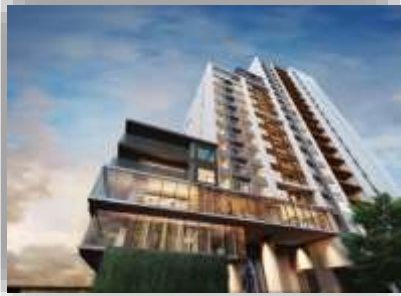
Parkland Charan Bored Piles
