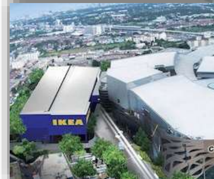
IKEA Westgate Bored Piles
