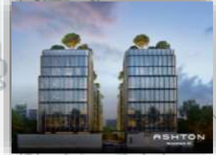
Asthon Residence 41 Bored Piles
