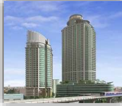
Le Luk Condo (A+B) Bored Piles
